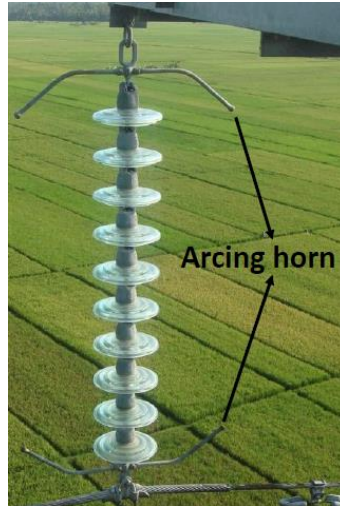
Gambar 14 Arcing Horn (PT. PLN (Persero), 2019)
