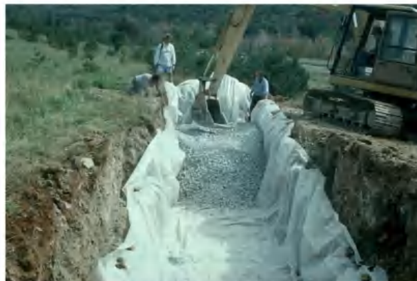
Gambar 8 Anoxic limestone drains / ALD (Skousen et al. , 2016)
