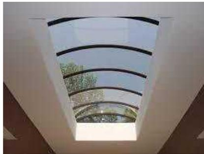
Gambar 2. 20 Barrel Vault Skylight
