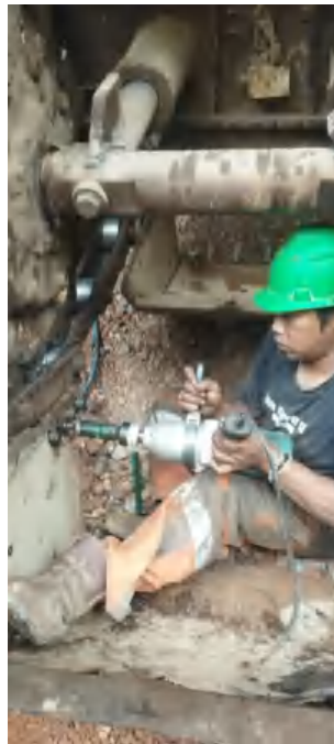
Proses penggantian part reclaimer clay
