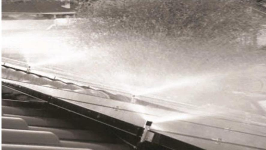
**Gambar 2** Sistem pembersihan air panel surya otomatis (Kazem et al., 2020)
