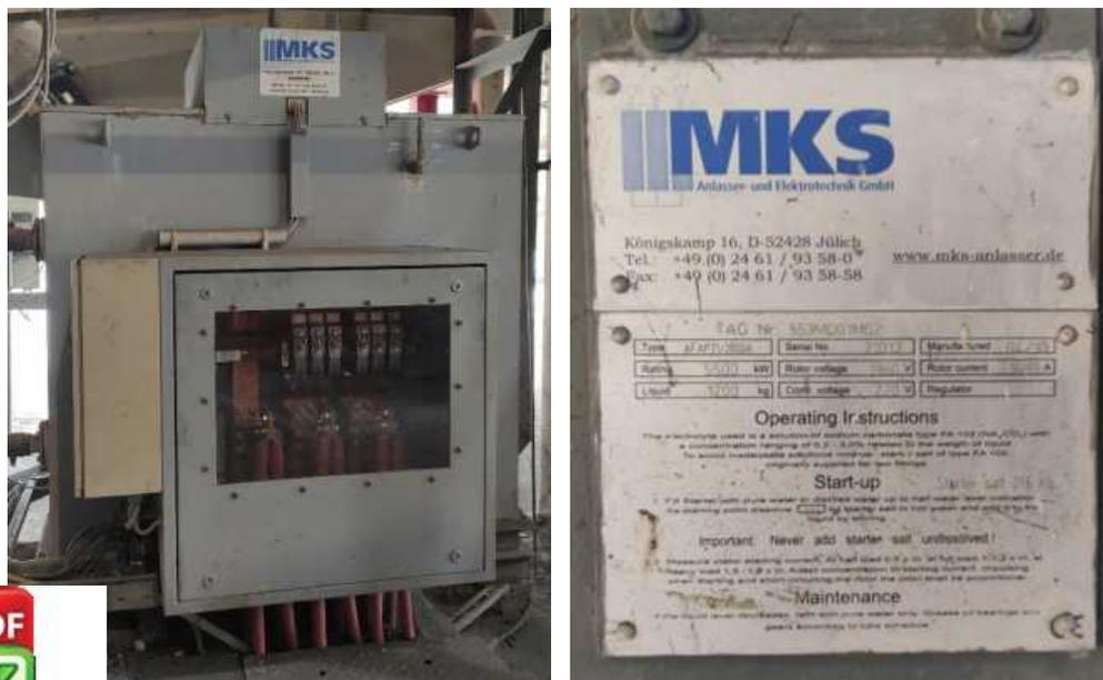
Gambar 17 Nameplate *liquid rotor starter*
