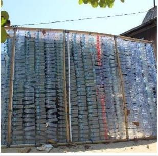
A photograph of a wall constructed from numerous discarded 1.5-liter plastic bottles, used as a research material.             |
