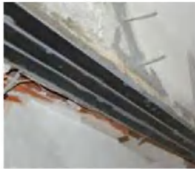
a. Bending reinforcement
