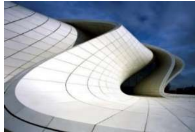
Gambar 2.178 Penggunaan Glass Fiber Reinforced Concrete (GFRC) dan Glass Fiber Reinforced Polyester (GFRP)
