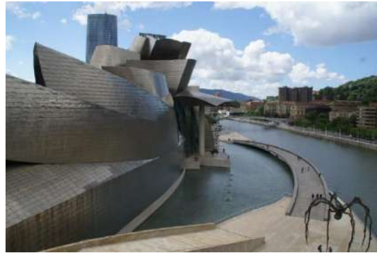
Gambar 2.94 Posisi bangunan Guggenheim Museum di tepi sungai utara pusat kota Sumber: https://www.archdaily.com/422470/ad-classics-the-guggenheim-museum-bilbao-frank-gehry
