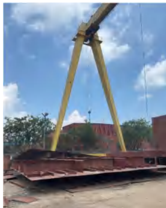
Gambar 1. Kegagalan Lifting Side Board
