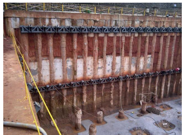
Gambar 12 Dinding Penahan Tanah Revetment
