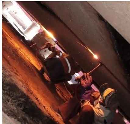
Gambar 5. Replating bottom Container Baruna Raya
