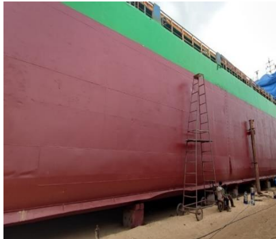
Gambar 2. Proses pengecatan Container Baruna Raya
