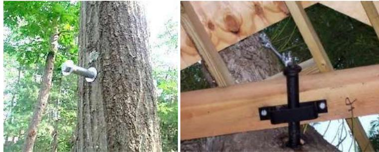
Gambar 12 Contoh Sistem Trees Attachment Bolt (TAB)
