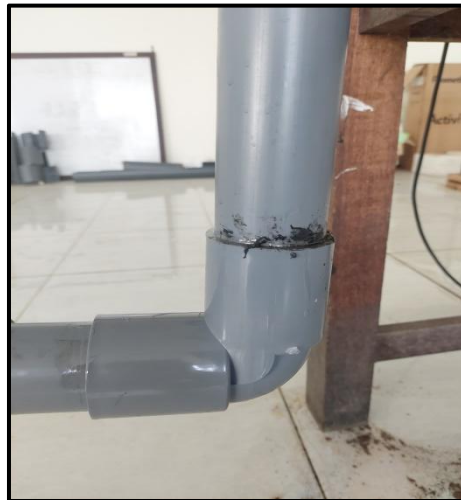
Gambar 29 Elbow 90° pvc 2 inch
