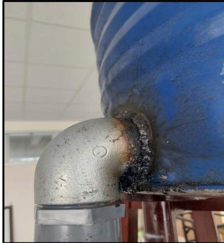
Gambar 30 Elbow 90° galvanis 2 inch
