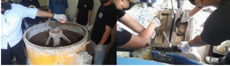
Lampiran 5. Pengecoran beton geopolimer
