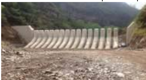
Gambar 4. Check Dam Tipe Slit
