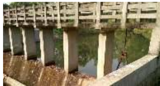
Gambar 3. Check Dam Tipe Beam
