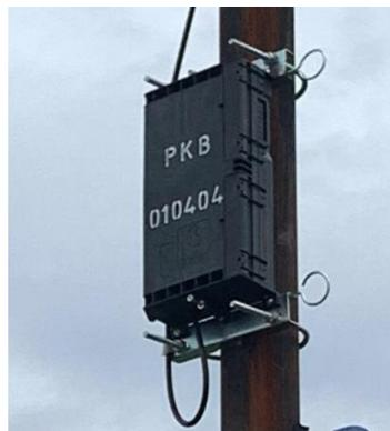
Gambar 5 ODP (*Optical Distribution Point*) (PT. Biznet)
