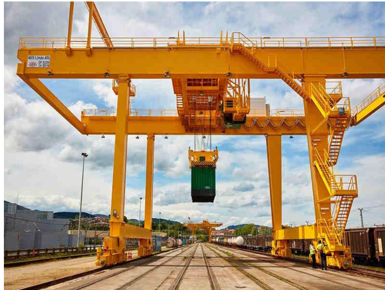
Gambar 2.5 Rail Mounted Gantry Crane (RMGC)
