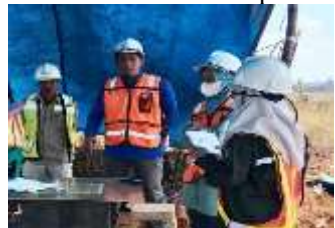
Observasi area Rehabilitasi
