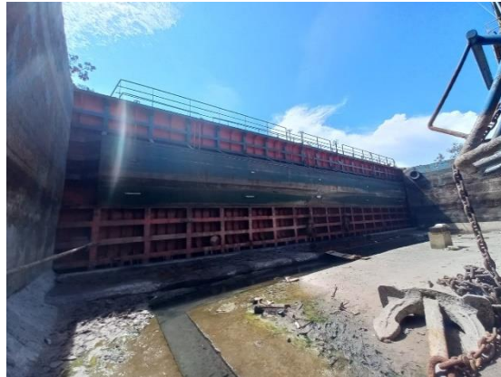
Gambar 2.2 Gerbang Graving Dock
