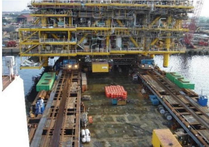
Gambar 2.1 Skidding System [2]
