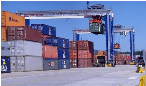
Gambar 17. Transtainer / Rubber Tyred Gantry (Sumber: airportassistant.wordpress.com )
