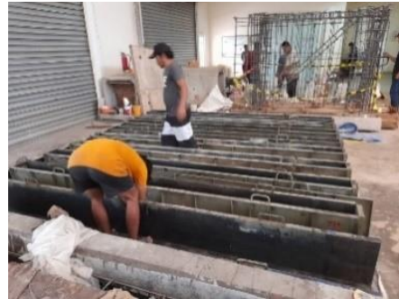
(b) Persiapan Bekisting
