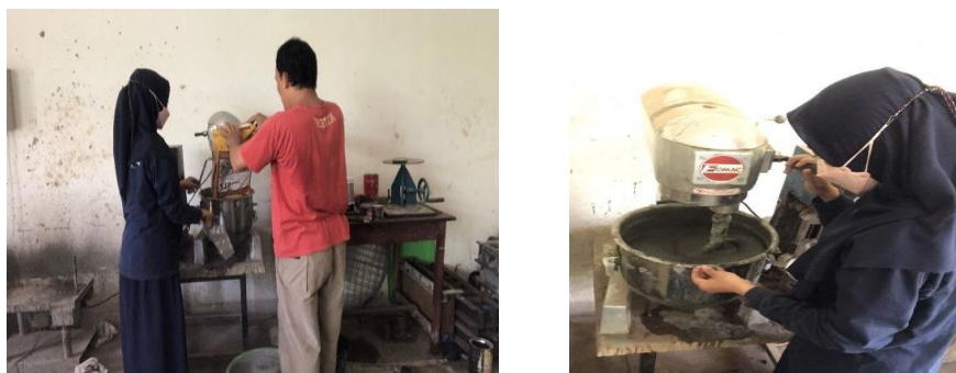
Gambar 32. Pencampuran Mortar Grouting
