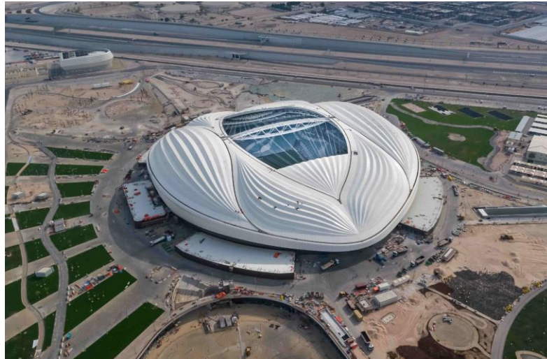
Gambar 12. Gambar Al Janoub Stadium
