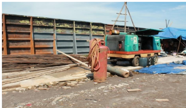
Gambar 1. Persiapan proses sandblasting
