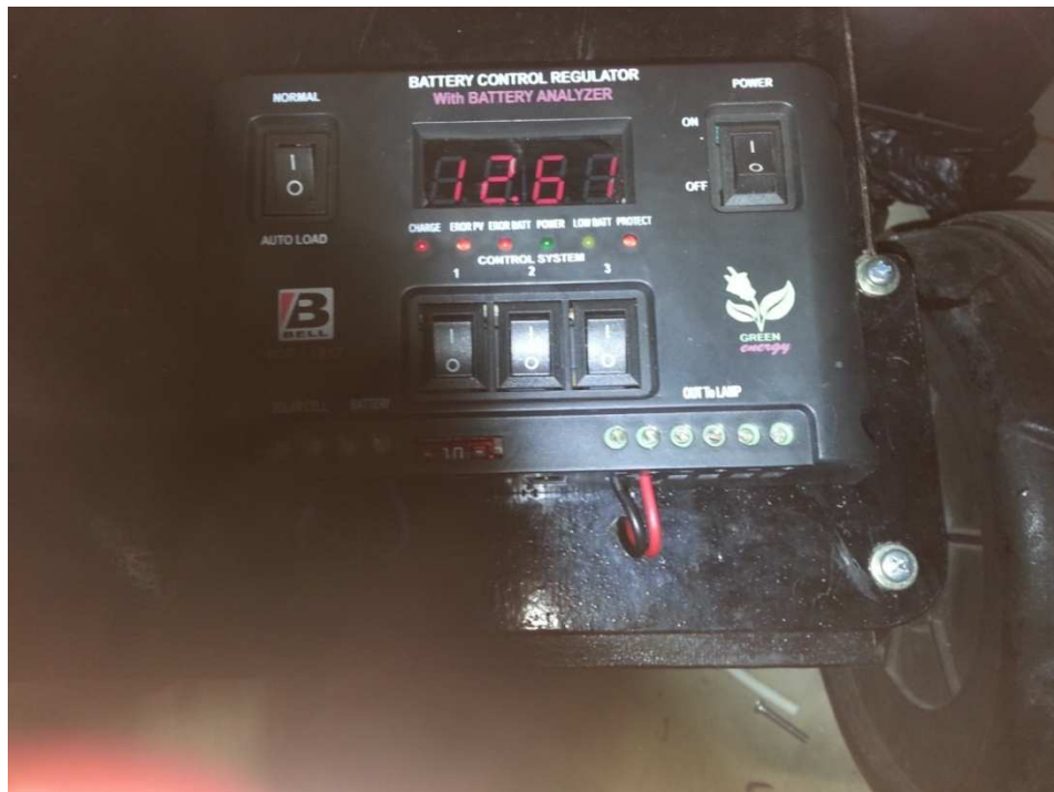
Pemasangan Battery Controller Regulator
