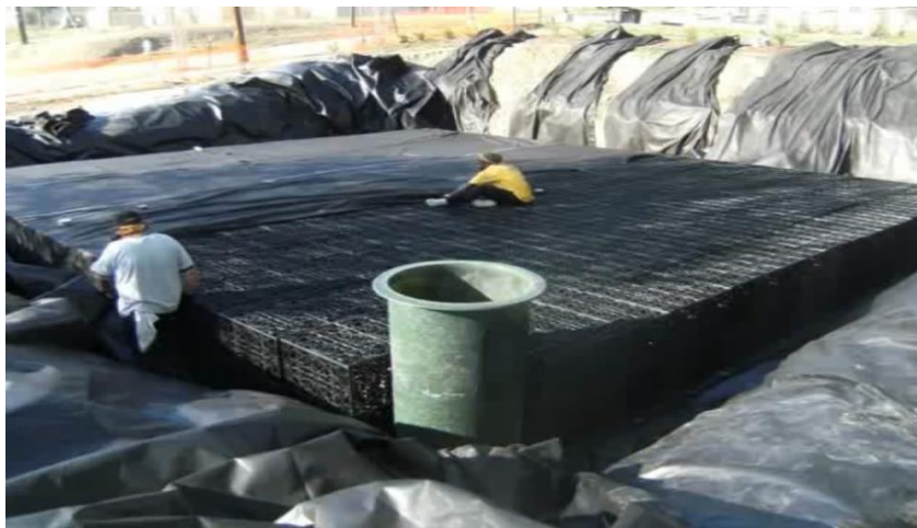
Gambar 2.8 Pemasangan Pompa Submersibel ( Submersible Pump ) kedalam volume penyimpanan Sumber: Video Youtube, Channel : Innovative Water Solution LLC, Dengan Judul “30.000 Gallon Modular, Underground Rainwater Harvesting | Innovative Water Solution”
