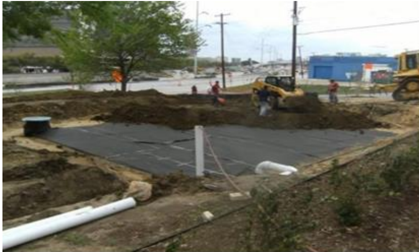
Gambar 2.9 Penimbunan Retention Tank
