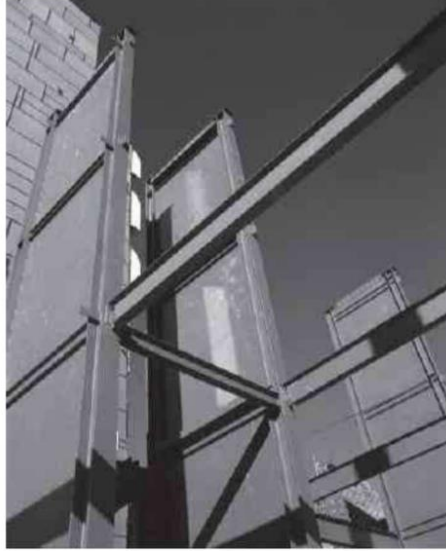
Gambar 14. SPSW di Canam Manac Group, Kanada ( Sumber: Richard Vincent, Canam Manac Group, Jl. George, Kanada)
