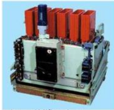
Gambar 2.1 ACB ( Air Circuit Breaker )
