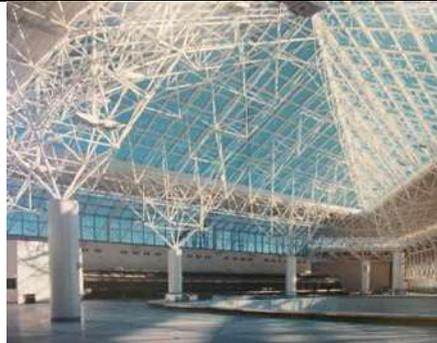
Gambar 10. Atap Rangka Baja
