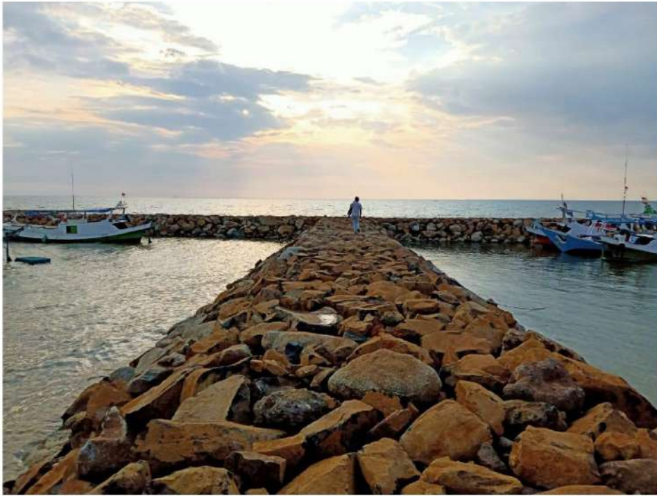
Tanggul Penahan Ombak (Groyne)
