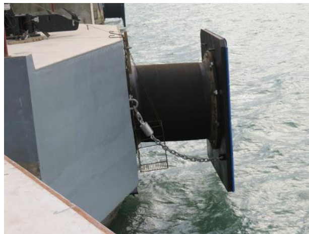
Gambar 2.5. Fender type sel
