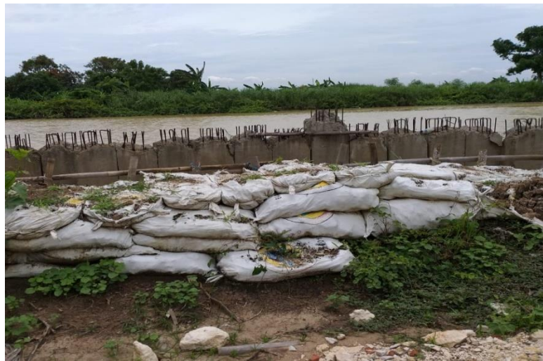
Figure 4.17: Existing embankments in the Muara Gembong area
