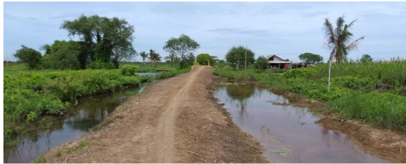
Figure 4.2: Access road in the Muara Gembong area
