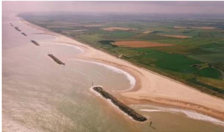
Gambar 5. *Detached Breakwater*
