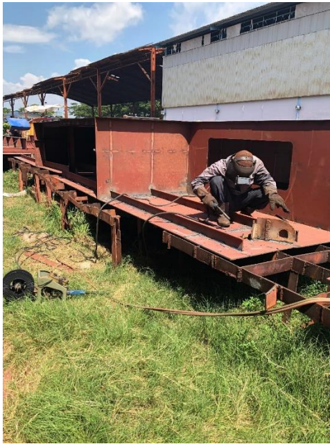
Proses Pengelasan FCAW
