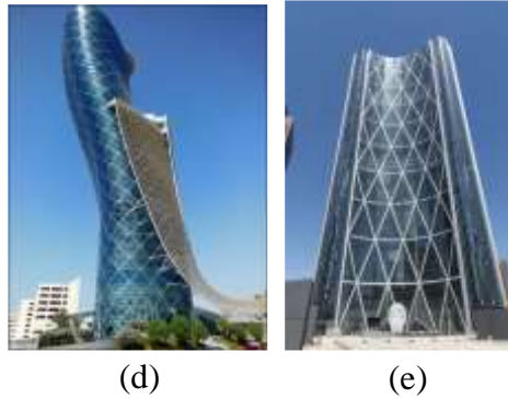
Gambar 14. (a) Swiss Re (b) CCTV Headquarters (c) Mode Gakuen Spiral Tower (d) Capital Gate (e) Bow Project
